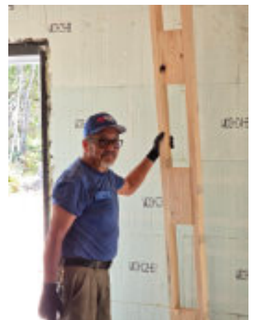
Raul Gonzalez doing interior framing.
