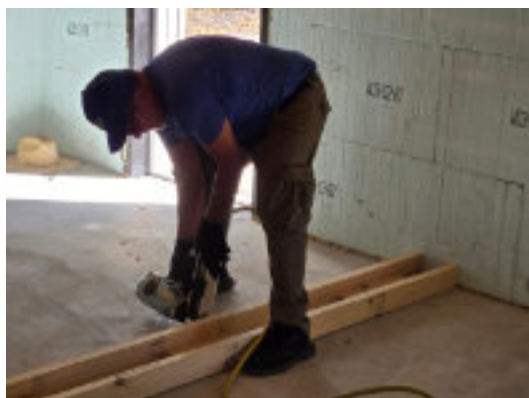
Raul Gonzalez using a nailing gun.
